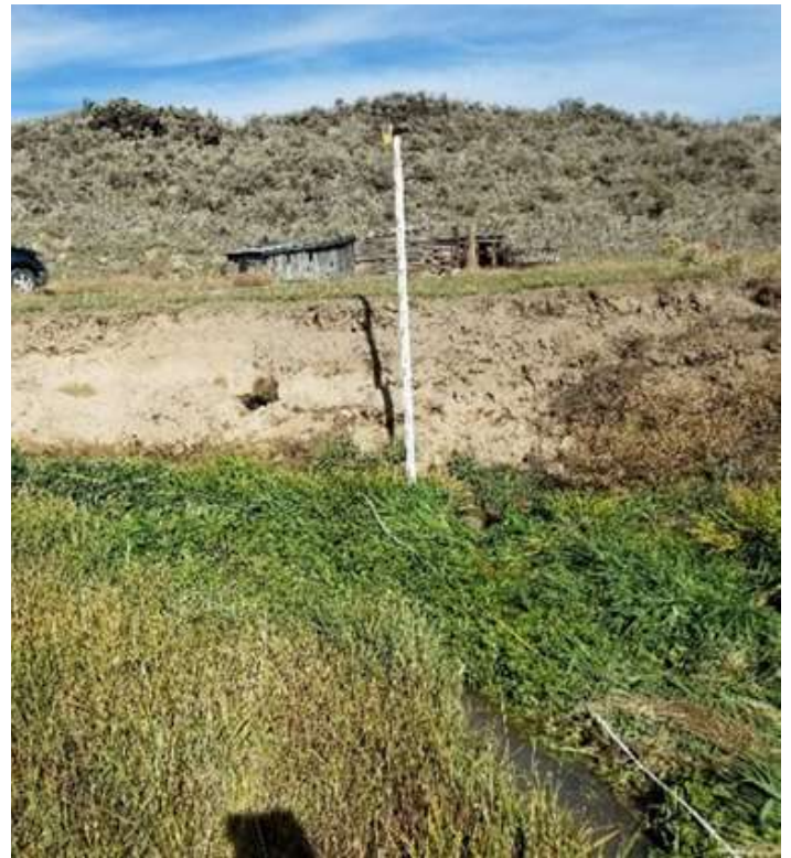
A measurement of the eroding bank on Cohn Creek
