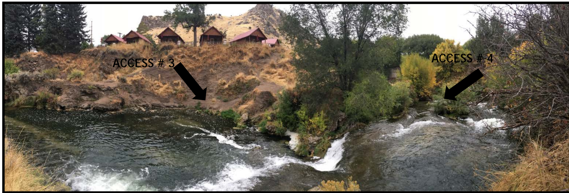
SOUTH VIEW OF COVE & ACCESS POINTS # 3 & # 4
