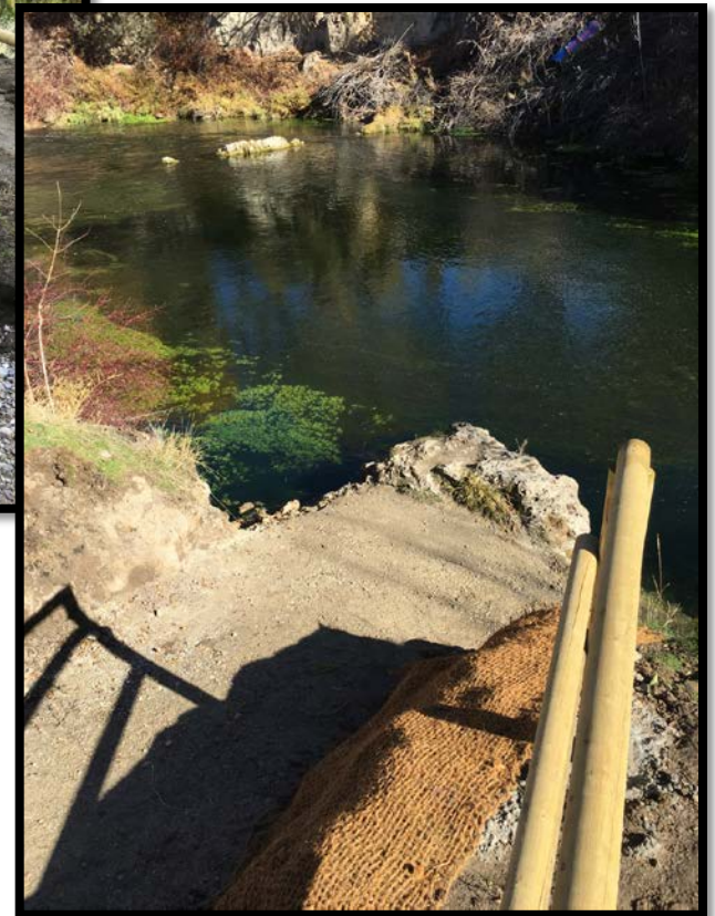
COMPLETED ACCESS POINT # 4
