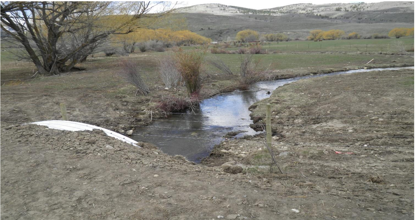
1 month after Stream Restoration, Pebble Creek South Channel-Riparian fence also installed.
